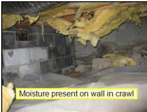
1.0 Picture 5 crawlspace under kitchen
