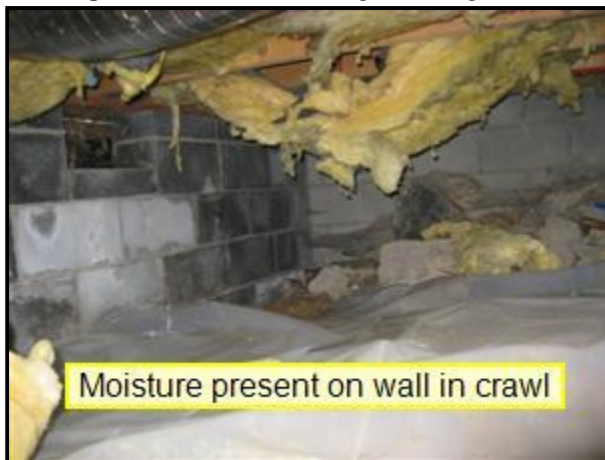
1.0 Picture 5 crawlspace under kitchen
