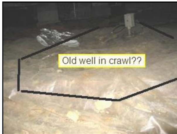
2.6 Picture 2 in crawlspace under new addition
