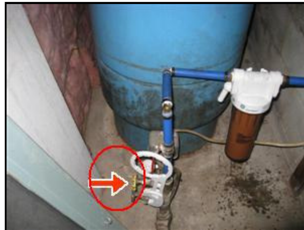
4.3 Picture 1 In basement
