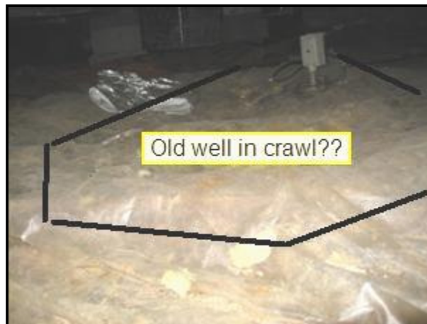
2.6 Picture 2 in crawlspace under new addition
